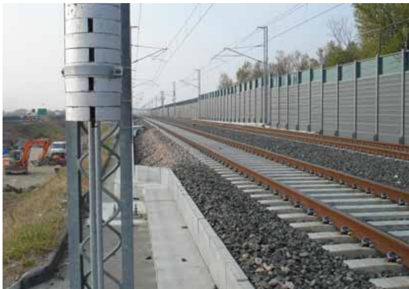
Fig. .... Panoramic view of the monitored section
