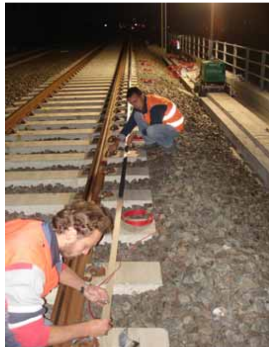
Installation of longitudinal RDS chain
