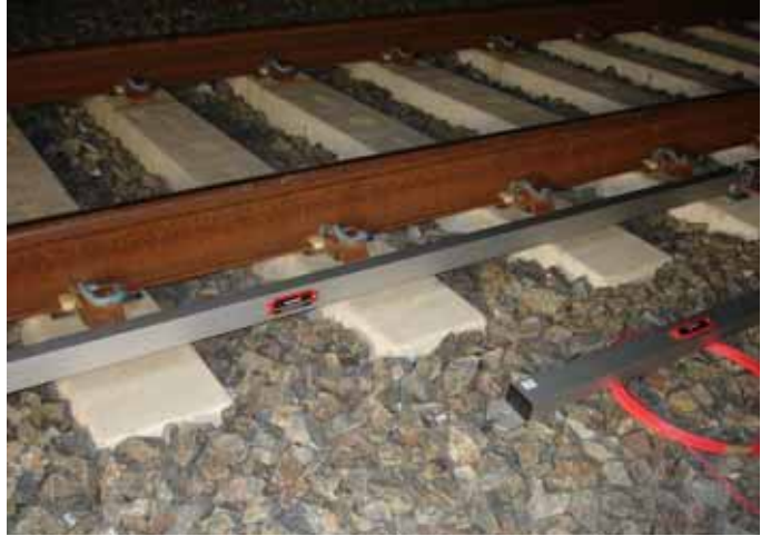
Removal of RDS longitudinal bars
