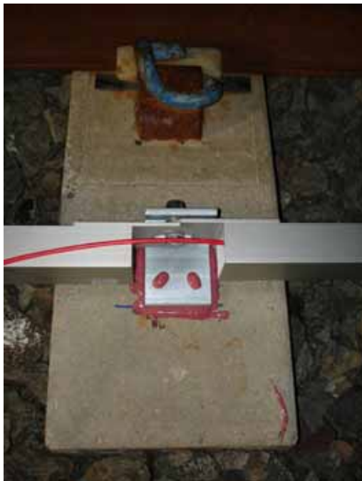
Installation of RDS longitudinal support by means of epoxy resins
